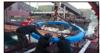
*The bearing is being pushed in place under the 2,500 ton crane.*
