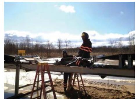
Figure 1. In addition to lock-out, tag-out, blocking the belt with engineered clamps and then confirming the conveyor cannot start is considered best practice.
